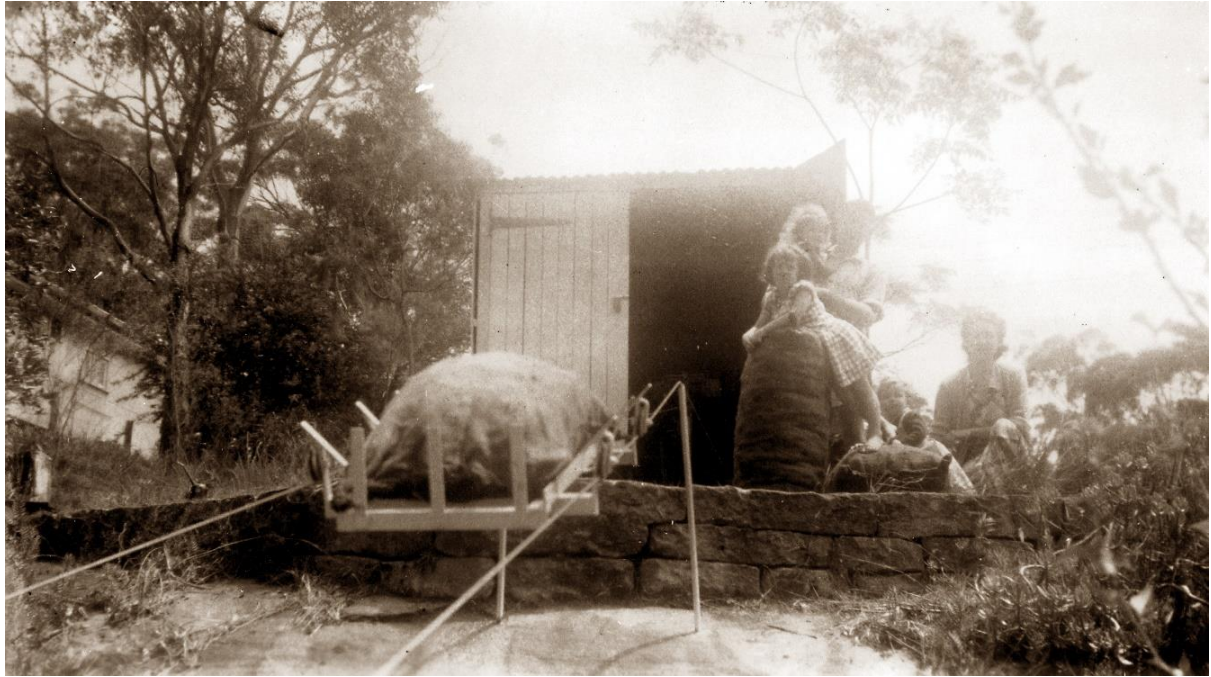
Figure 6.3 The cable-pulley system that moved bags of oysters from the waterfront to the top of the embankment, with members of the Matthei family shown near the engine shed behind. The cable-pulley engine shed remains on the site. (Source: Linda Henderson)
